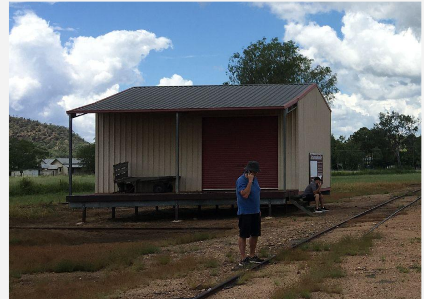
Picture 11: Railway shed @ Dupre
