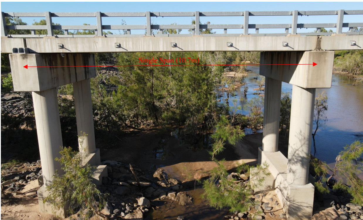
Photo 3 – Northern View of Bridge (single span)
