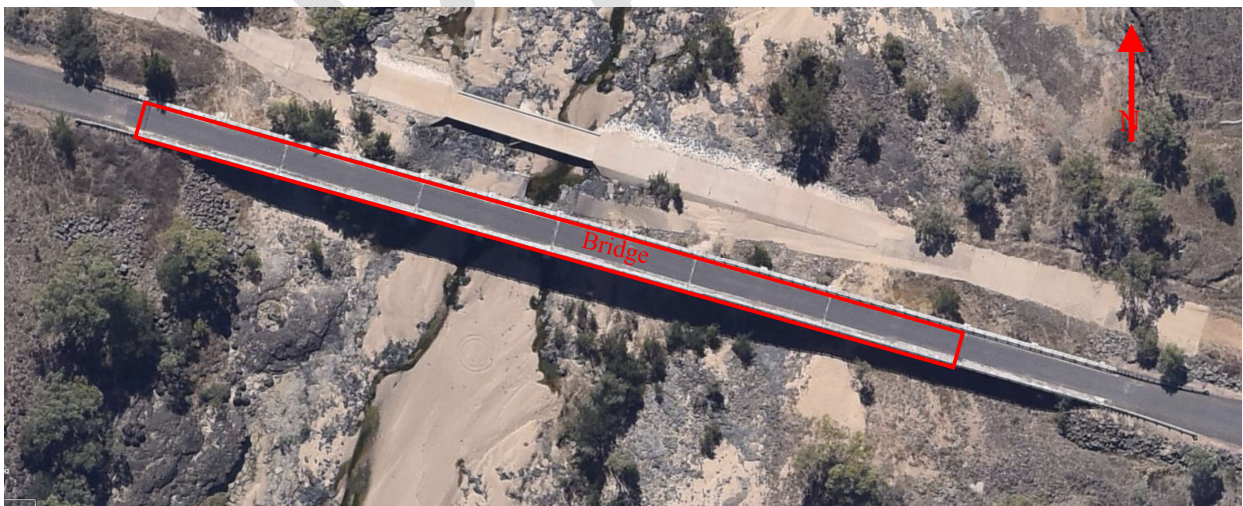
Photo 1 – Aerial view of location over Copperfield River
