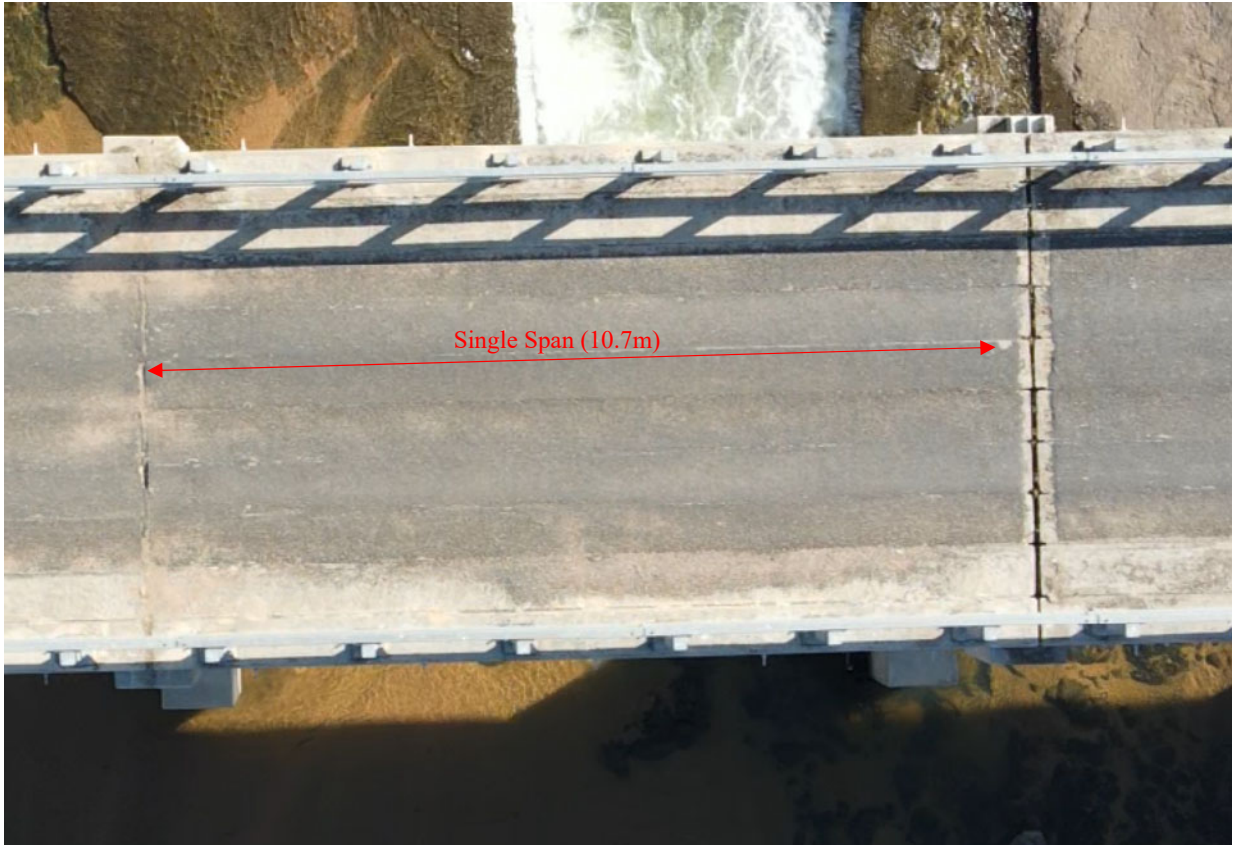
Photo 2 – Single span of bridge
