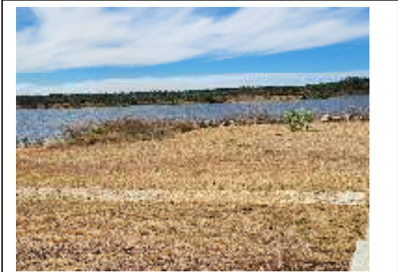
Photo 13- Charleston Dam – Facing South
