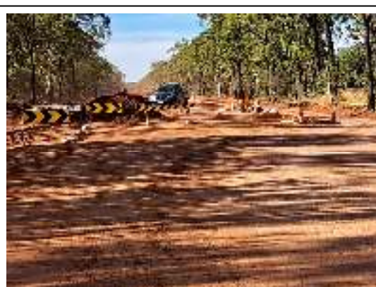
Photo 8 – Facing East – Ready for road base Einasleigh - Forsayth Road
