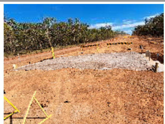
Photo 9 – First structure (3 cells box culvert) Einasleigh - Forsayth Road
