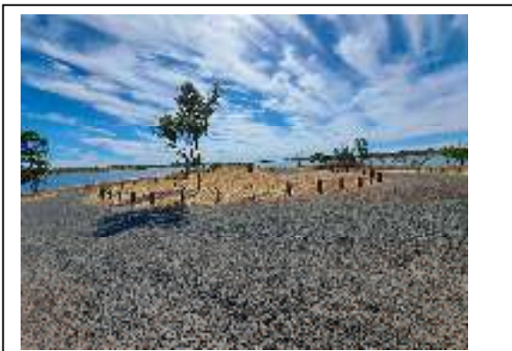
Photo 12 – Charleston Dam – facing East
