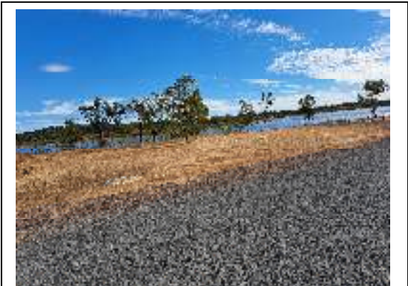
Photo 15 – Charleston Dam – Facing North
