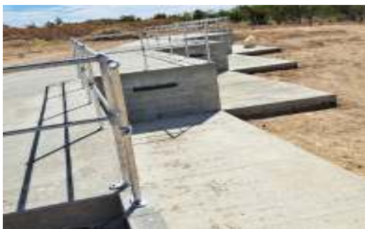
Photo 3 – Bin Concrete slab
