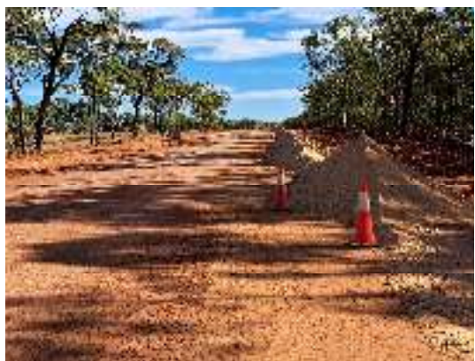
Photo 7 – Facing west – ready for road base Einasleigh - Forsayth Road (75 % completed)
