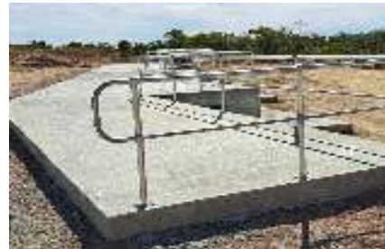
Photo2 – Facing East North ( Concrete structure detail )
