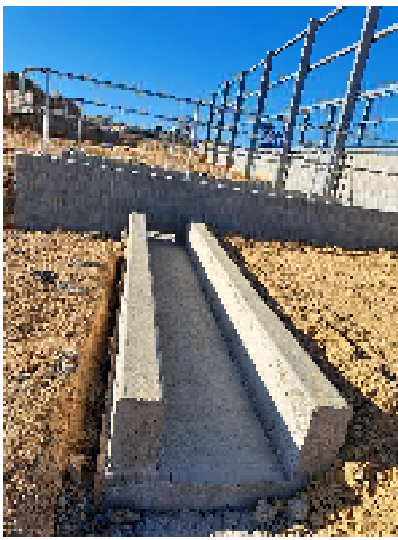
Photo 3 – Facing East – Effluent access channel
