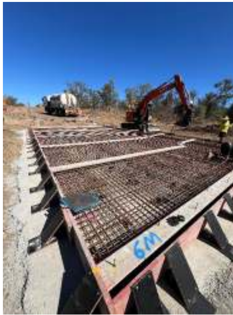
Photo 6 : Slab reinforcement
