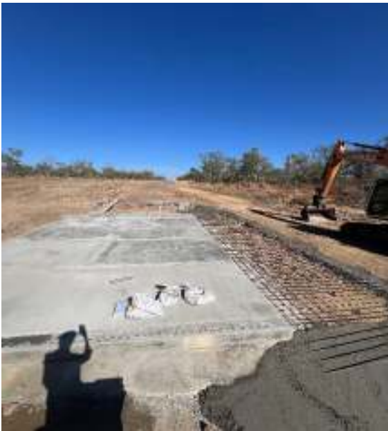
Photo 5: Facing North (Concrete slab and d/s cut off wall)
