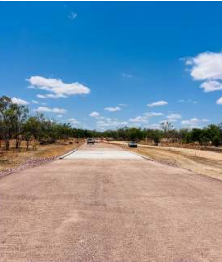
Photo 1 : Facing South West
